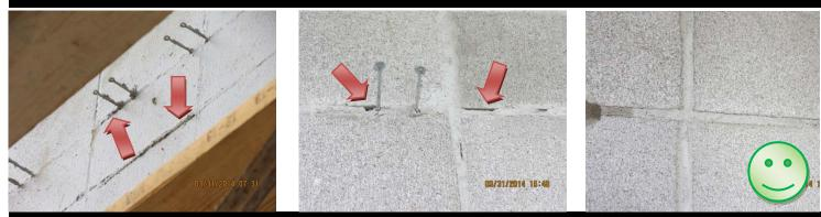
Discuss the masonry joints...They need to be full, properly tooled (<u>compressed</u> in the joint, either flush or concave)...We do not want the joints to have voids or mortar sticking out of the joint, creating ledges and improper membrane thicknesses at these irregular shapes, potentially creating failure in the AVB system.
